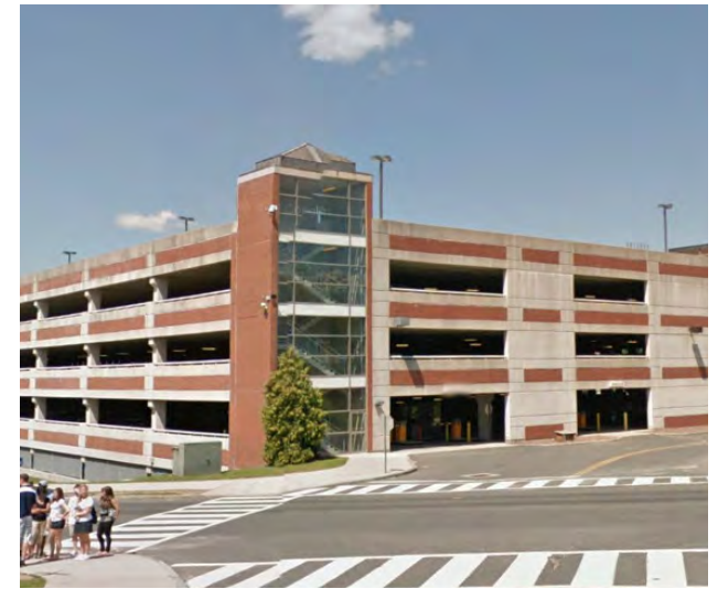
North Parking Garage
