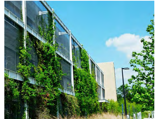
Living Garage Facade: National Wildlife Federation Headquarters, Reston, VA
